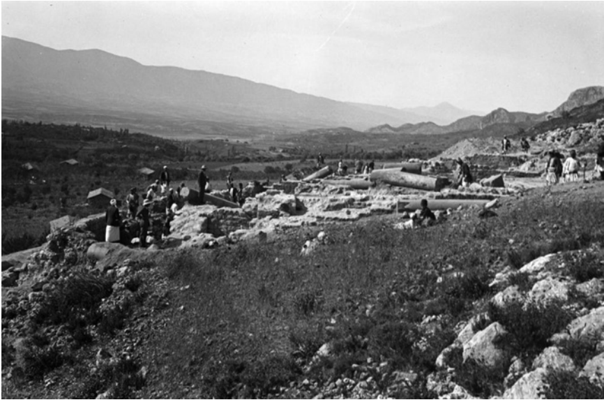
FIGURE 6.9 D-53-J/K, Church at Daphne, general view of excavations, looking north
